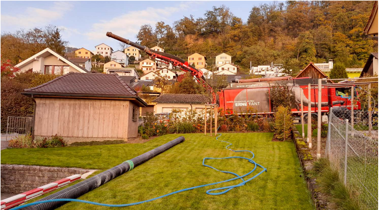
Reparatur in Klingnau
